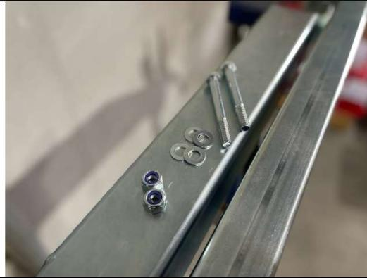
Place the upright between the loose side plates. Install the top bolt with washers on either side. Loosely attach the nut.
